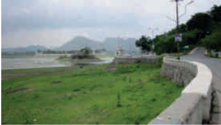
Lake Fateh Sagar, Original Stone Banshi being replaced by new replica of the same.
