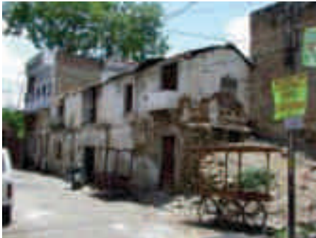
view of dilapidating historic fabric in residential street at Kanji Ghata
