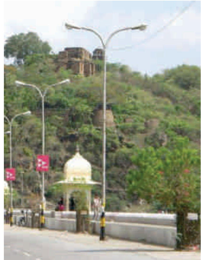
The structures on Moti Magri in need of attention
