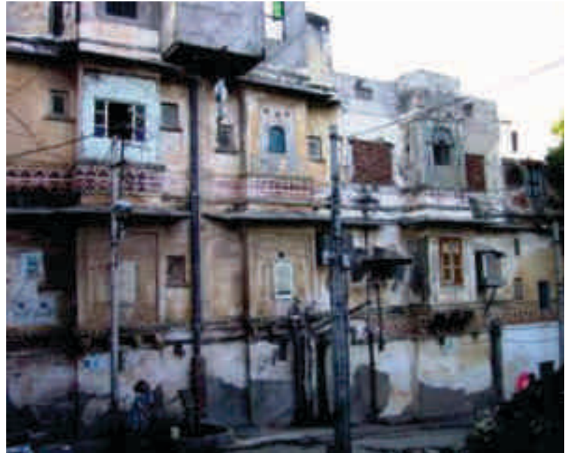
A view of the Mammayon ki Haveli – the interventions can be seen as added projected block on the third floor, alteration of original openings and repairs in cement and brick infill, reflecting lack of awareness towards heritage conservation
