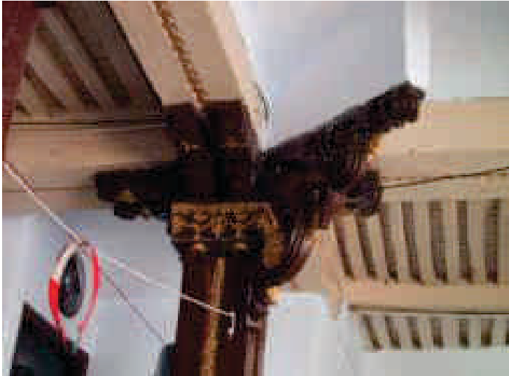
Haveli at Salumbher with use of timber as structural members.
