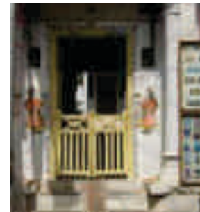
Typical door detail of a house accessed from the street. The wall painting around the door frame and on the sides are common feature till date with the traditional styles of painting thriving.
