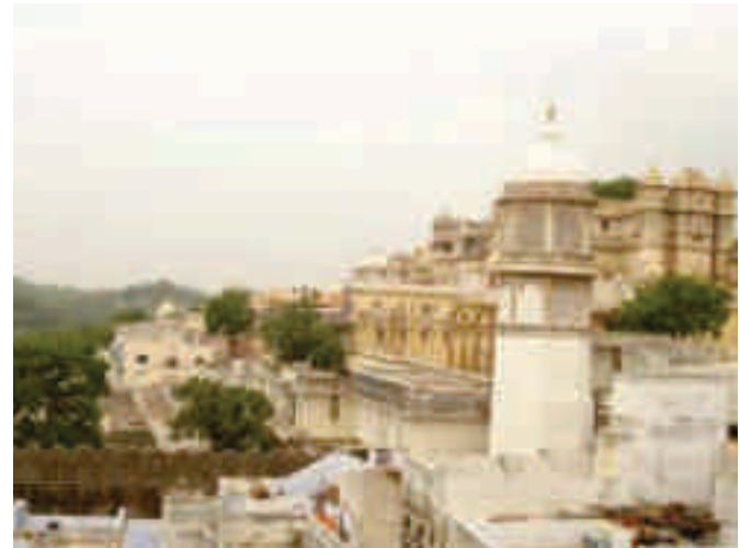
The City Palace Complex, Udaipur
