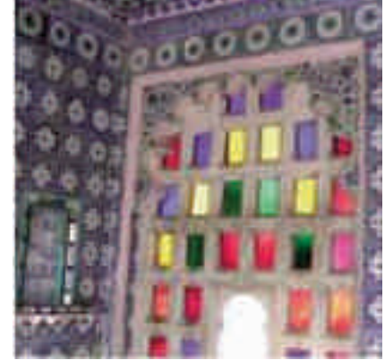
Glass inlay, stained glass, china tiles set in lime mortar, City Palace, Udaipur
