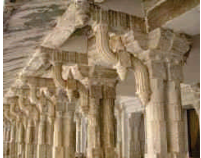
Seven foot wide stone sunshade supported by carved stone brackets and columns, City Palace, Udaipur.
