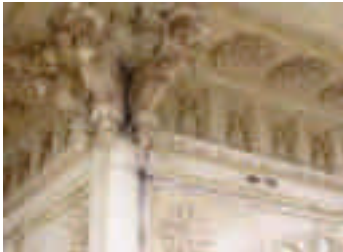
Stone carved members in the City Palace Complex, with araish plaster
