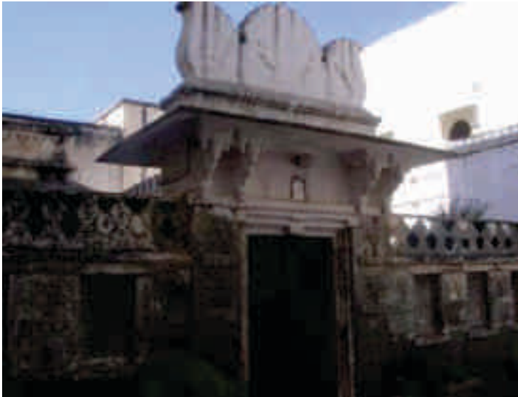
Poorly maintained though intact structure before restoration
