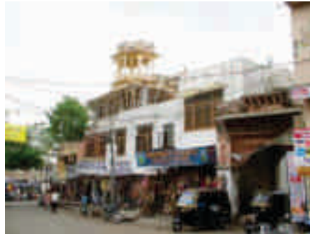
view of commercial street from Tripoliya gate of the City Palace to the Jagdish temple Chowk shows a dilapidating historic gateway and new construction of a framed structure in reinforced cement concrete being carried out
