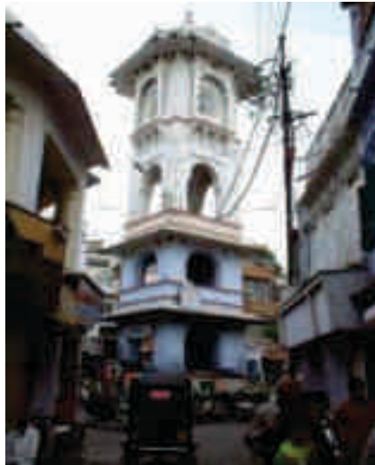
Electrical cables extending in to the Clock Tower/ GhantaGhar – a threat to the historic structure with regards to fire safety
