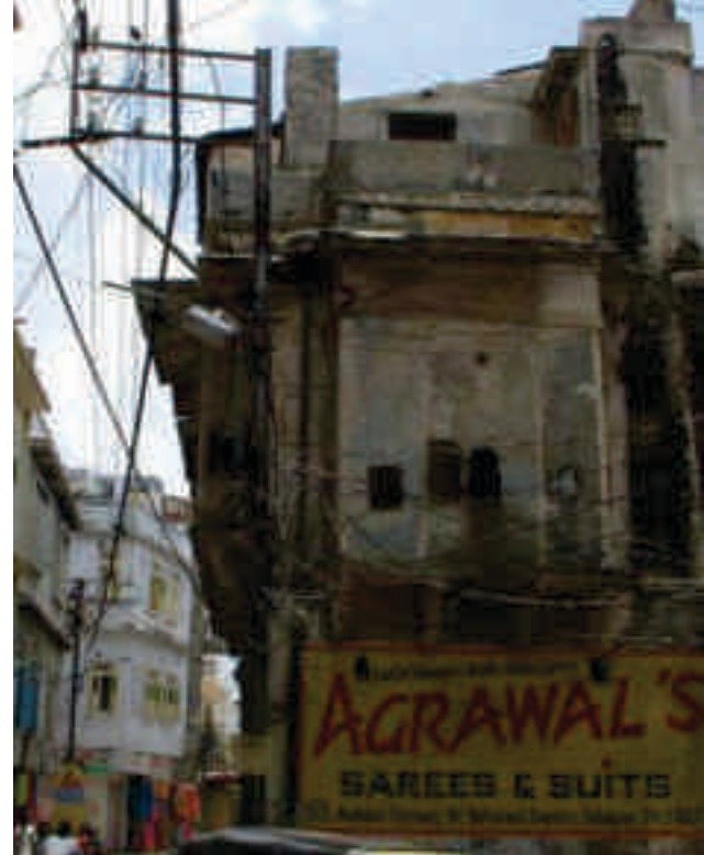
The inner lanes with unorganised electrical cables wires and fittings and narrow width make them high risk with regards to fire safety
