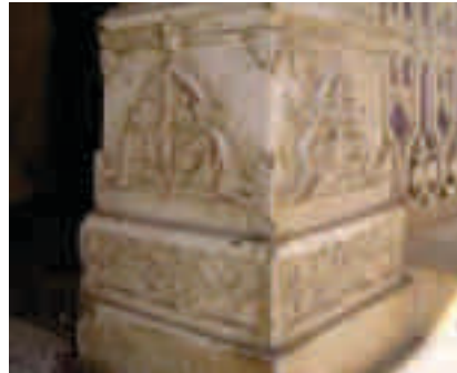
Typical stone column base with araish (slaked lime smooth finish) finish, City Palace, Udaipur
