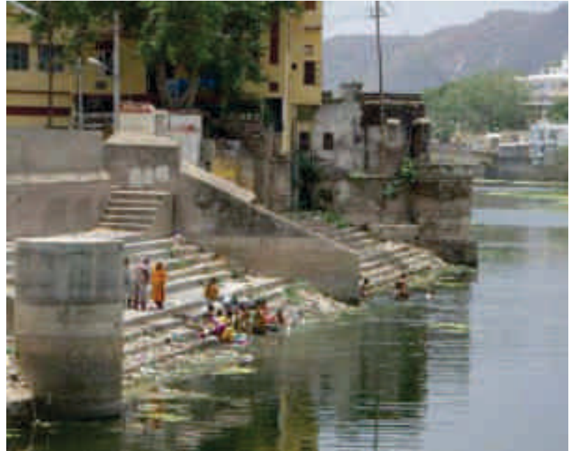
The ghats of Swaroop Sagar being used for bathing and washing of clothes and for dumping of solid waste and sewage causing contamination of the water
