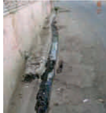
Open drains along streets in the walled city carry storm water, sewage and sillage in the absence of an efficient underground sewerage system.
